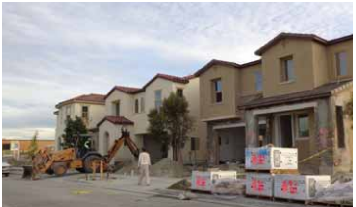
Ridgewood model homes under construction
