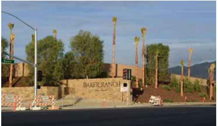
Baker Ranch entrance from Bake Parkway
